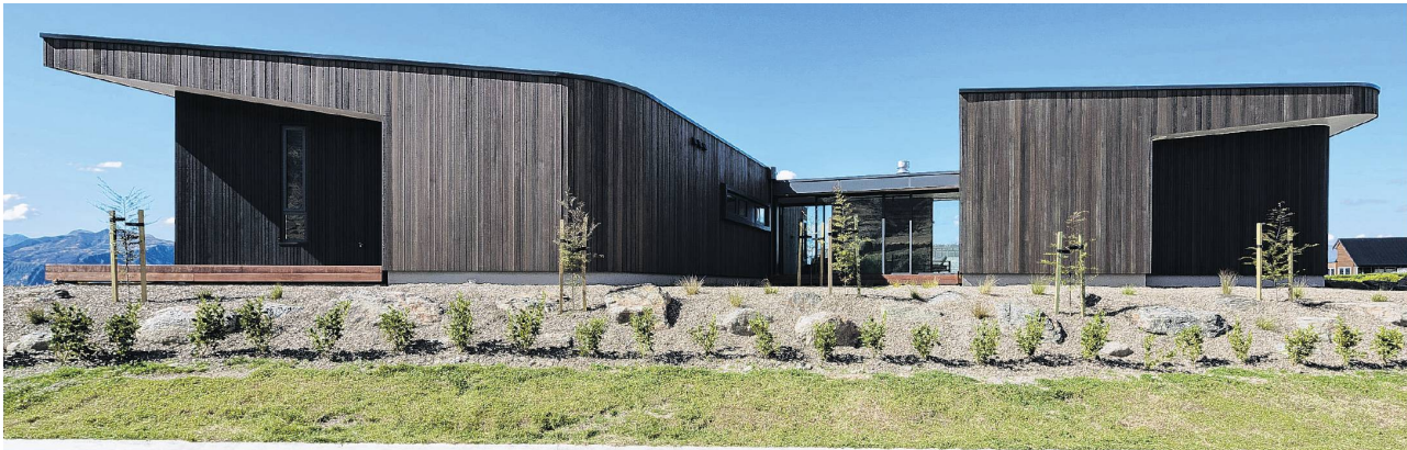
Two types of cedar cladding, with a dark and a warm stain, accentuate the lines of the windows and roof of this Wanaka home, designed by Condon Scott Architects.
