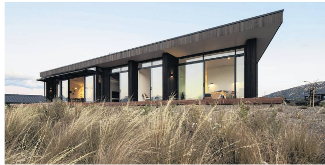
The mono-pitched roof directs the eye out to the lake and the mountains.
